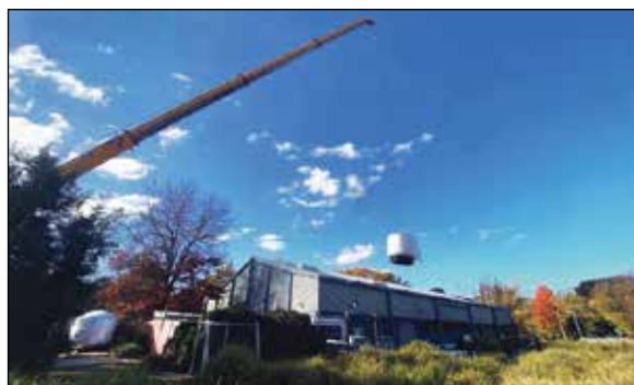
The new filter system is put in place using a crane.
