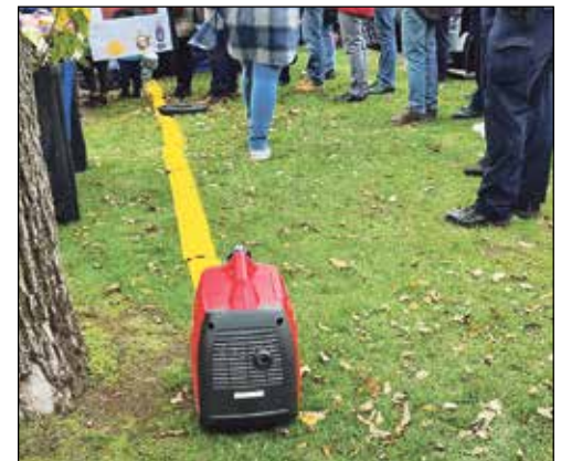
The RSL's generator provides power to the Gisborne Anzac Day service in April.
